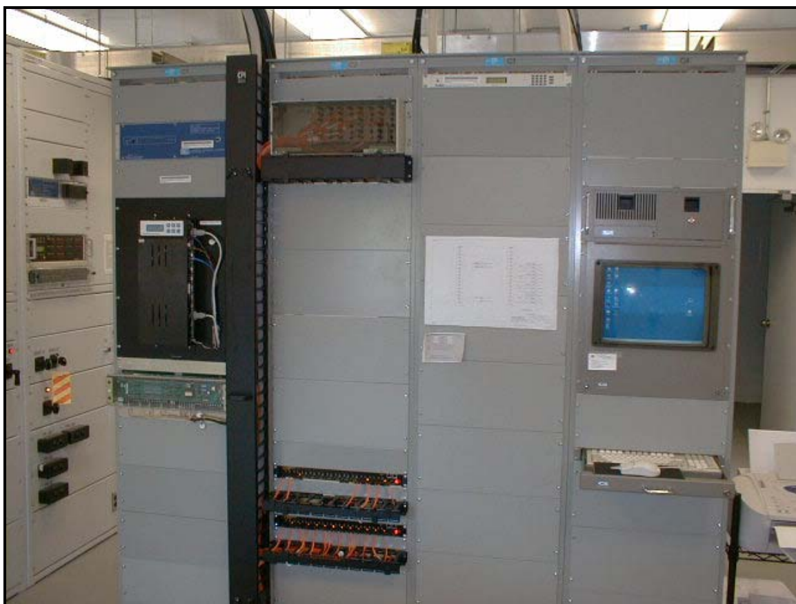
Figure 5 – Siemens Stationmanager, Station PC, and Network Components
