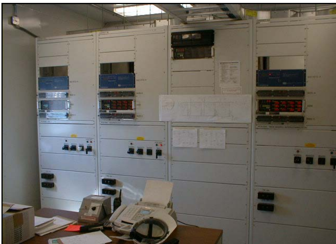
Figure 6 – Cooper EdisonPro and SEL-321 Relays
