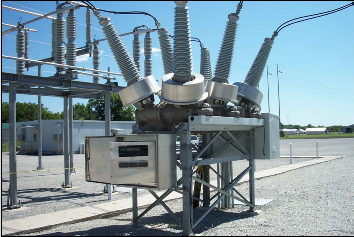
Figure 7 – GE D60 Relay located in cabinet at Siemens 161kV Circuit Breaker
